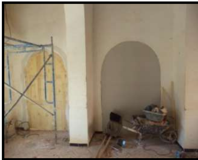
Figure 11: Image showing the position of the arches after the intervention
