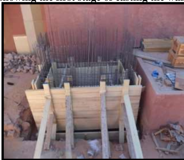
Figure 12: Picture showing the first stage of casting the wall of the water tank.
