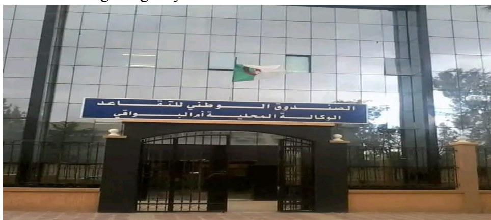
Fig.1. Front Facade of the National Retirement Fund (CNR) – Oum El Bouaghi Agency
